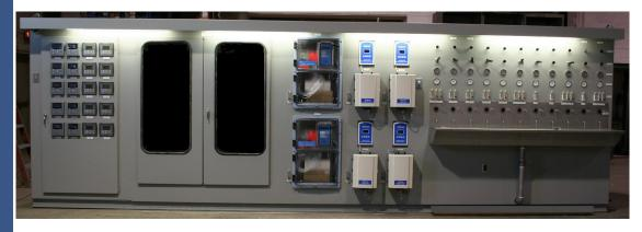
To monitor and maintain proper chemistry within the process by taking samples to analyze for levels of pH, conductivity, silica, sodium, solids, chlorine, DO, TOC, etc.
